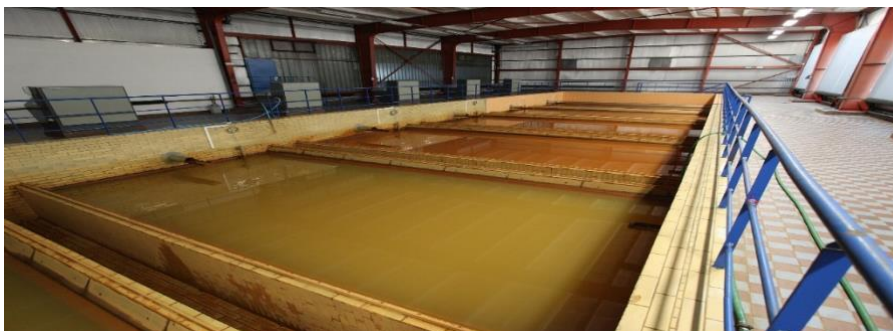
“Tanks with sand filters to remove precipitated iron (not working at the time)”
