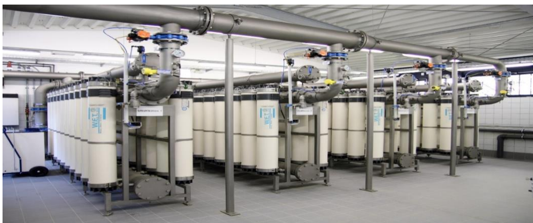
“Drinking water treatment of 300 m 3 /h using ultrafiltration in Grundmühle waterworks (Germany)”
